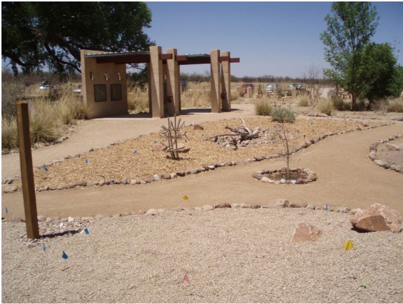
A xeriscape employing both gravel and bark mulch and accented with boulders, river rock, and branches. Note the use of multi-colored flags to denote the location of a buried 1/2" drip line and where to place plants.
