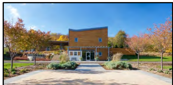
Renovated Granary is now the Visitor Center shown with conversation patio with Cherry trees and perennial beds
