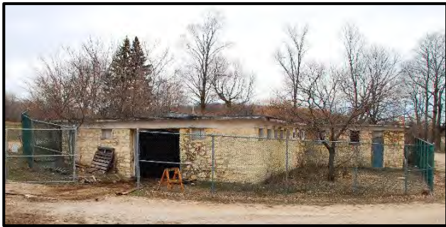
Old horse barn stone foundation before the Walled Garden was established.
