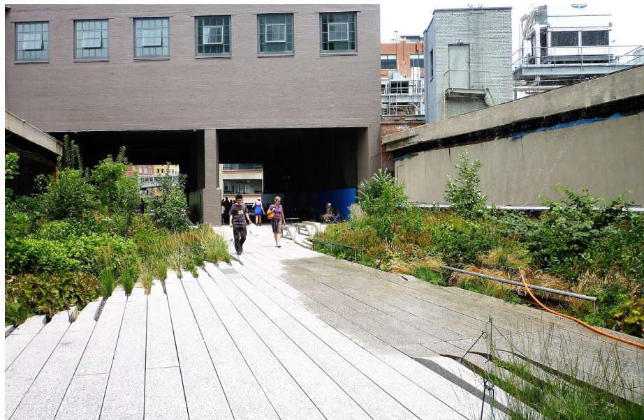
▲ Grasses grow up through the tapered edges of walkways.
